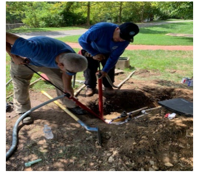
Irrigation repair at Brenman Park.
