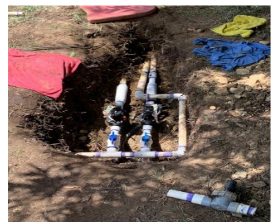
Irrigation repair at Brenman Park.
