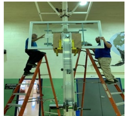
Backboard installation/replacement at John Adams.
