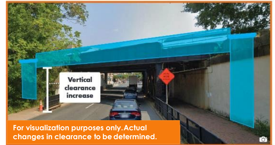
King Street looking east. The proposed recommended design option will increase the vertical clearance underneath the railroad bridge.
