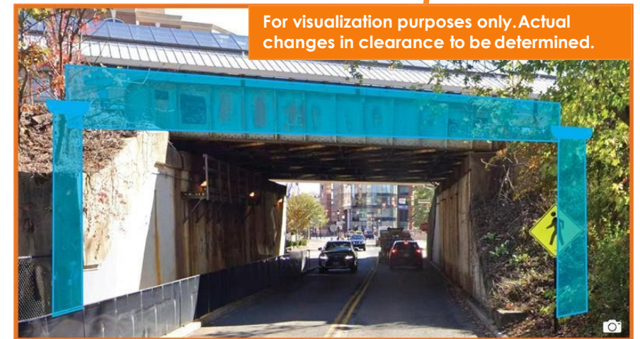
Commonwealth Avenue looking east. The proposed recommended design option may increase the horizontal clearance underneath the railroad bridge.
