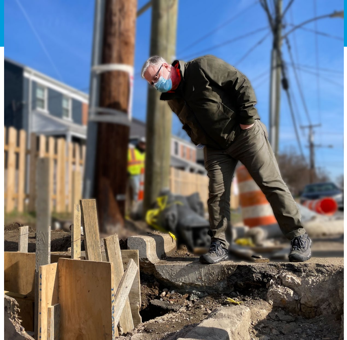
Engineer Brian Rahal, of the Stormwater Management Division, monitors progress on larger inlet installation on Hume Avenue on Jan. 24, 2022
