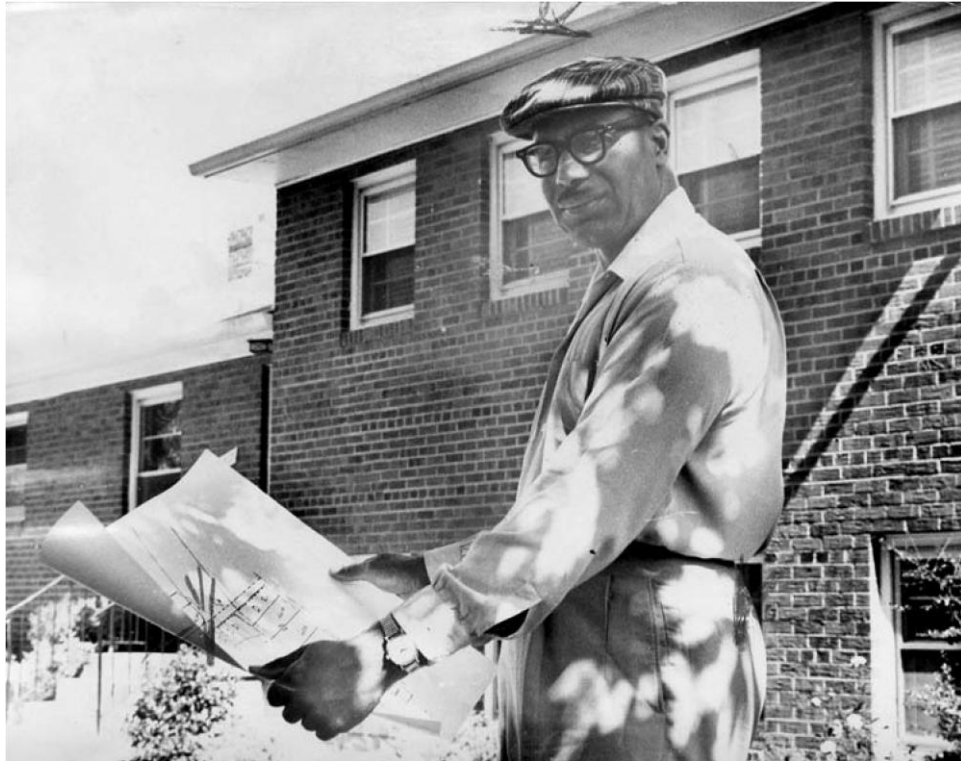
Marion Johnson looking at plans for the newly built Seminary neighborhood in 1962 ( Special Collections, DC Public Library )
