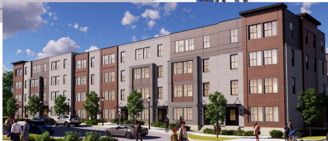
Figure #3: Front Façade of Stacked Townhouse CO#2
