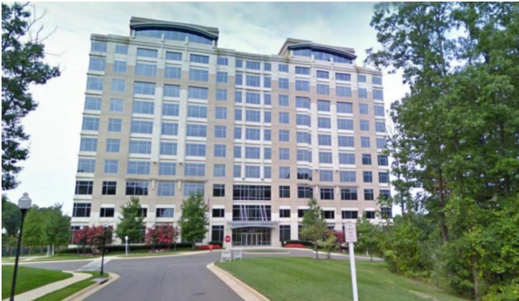
Exterior of building – 4850 Mark Center Drive
