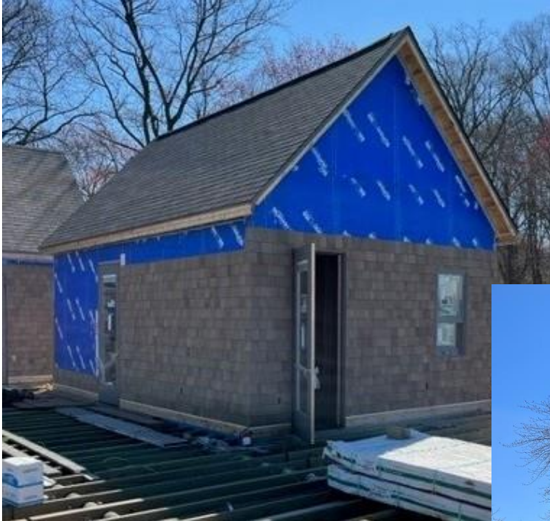
Gift Shop Shingles & Roof
