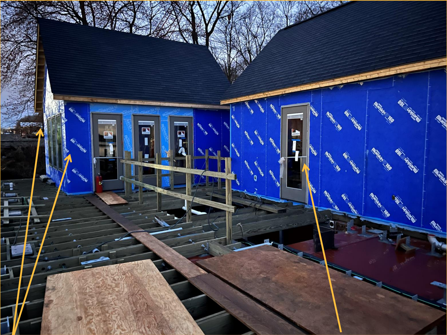
Education Center Doors & Windows; Naval History Theater Door
