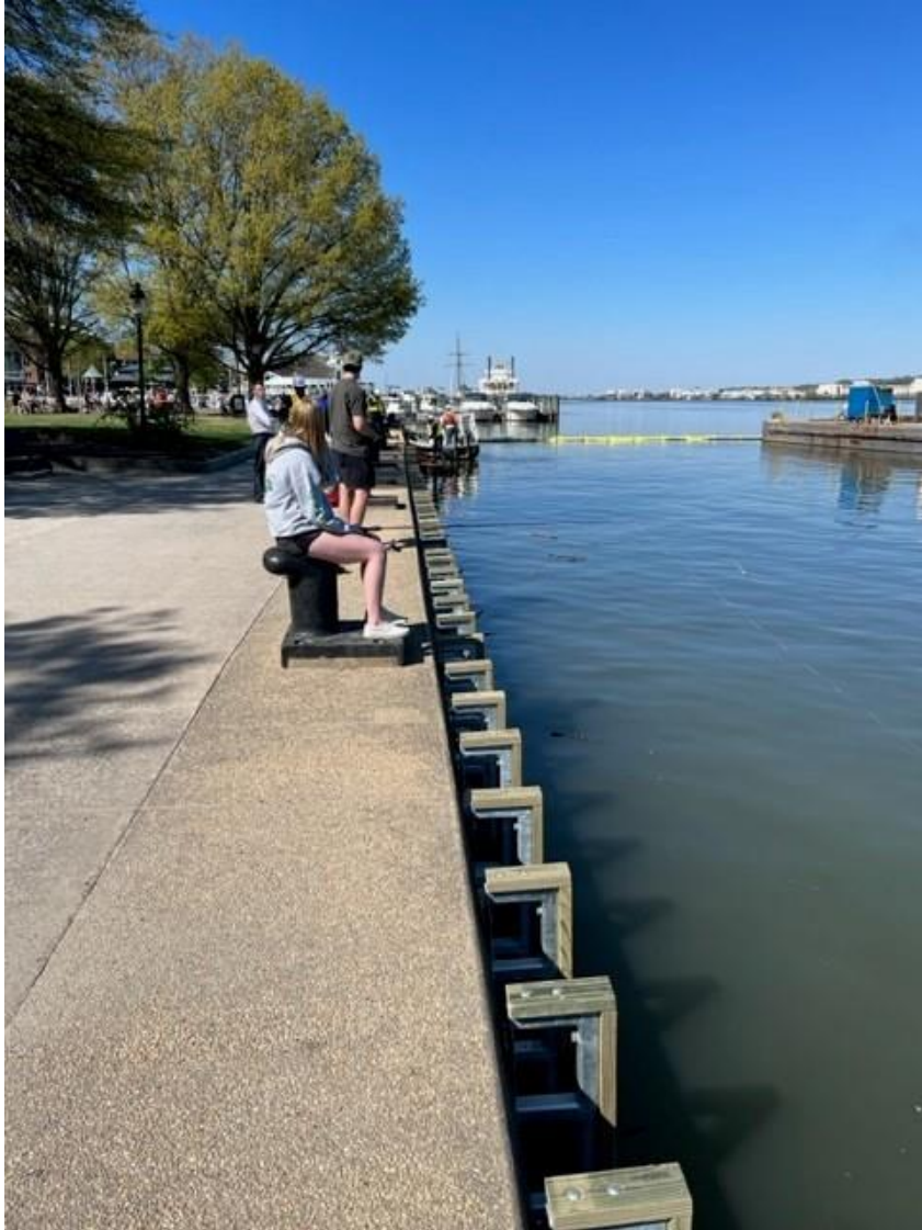
Brackets for utilities
