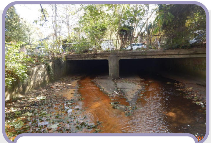
Hooffs Run Culvert at E. Linden Street under dry weather conditions.
