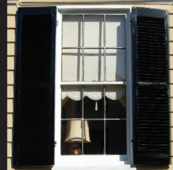
^ 6/6 FEDERAL / GREEK REVIVAL
