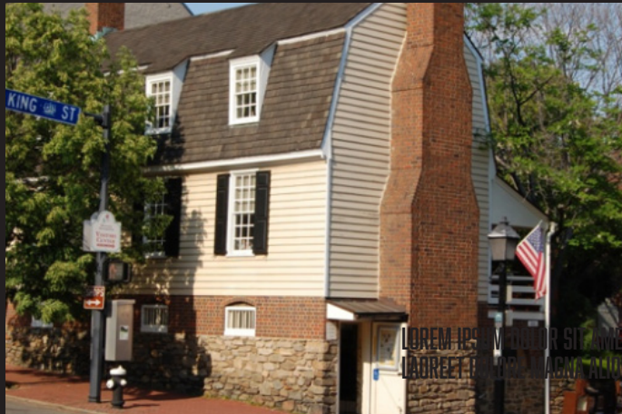
The now exposed stone foundation of the 18th-century Ramsay House shows the original height before King Street was regraded in the early 19th Century.
