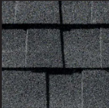
^ ARCHITECTURAL GRADE ASPHALT 20TH - 21ST CENTURY
