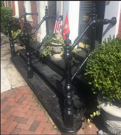
Example of historically appropriate cast iron steps and handrail on an Italianate style residence.
