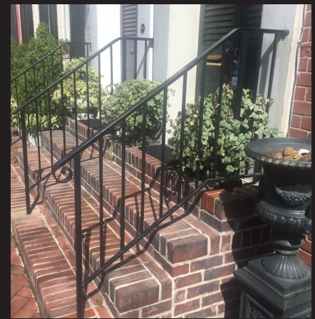
Example of inappropriate modern brick stoop and iron handrail on an Italianate style residence.
