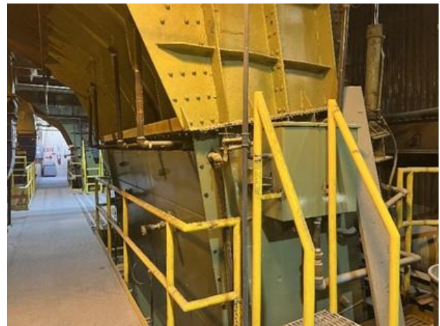
Photo: New feed chute on Boiler No. 2.
