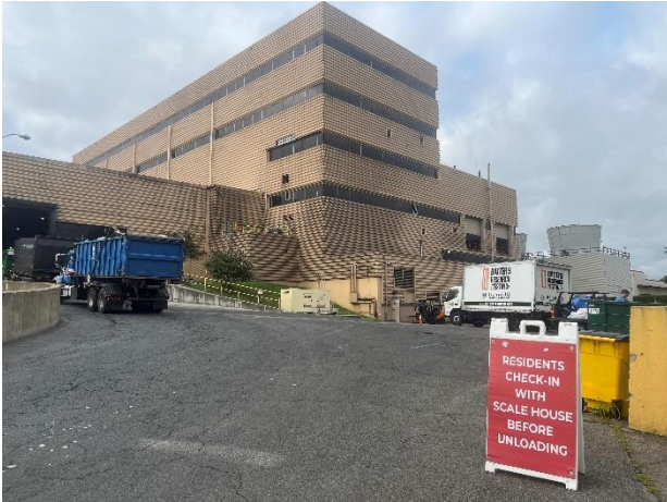
Photo: North side of Facility.
